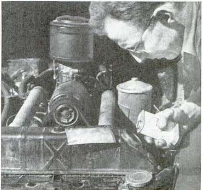
Clean spark plugs and proper gaps aid efficient engine performance. Above, inspecting plug for oil and gap measurement
